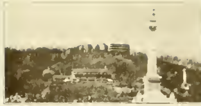
CRAVENS HOUSE AND POINT HOTEL. LOOKOUT MT.
